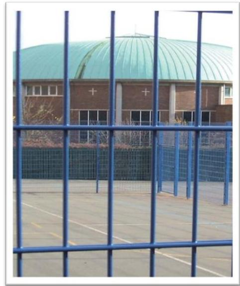
**Duo Panel option.** As with the 'multi-mesh' system, the Bastion Duo Sportsfence is available in heights of 3, 4 and 5mtr. The Bastion Duo panels are manufactured from 6mm vertical wires and twin 8mm horizontals
